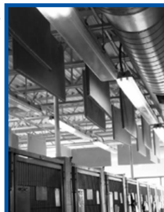
The new sound baffling in our dog kennels. Thanks to all the donors at the Dog Ball who made this possible!
