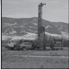
Digging one of the wells on the site.
